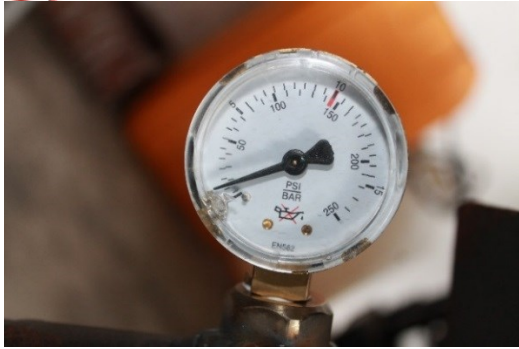
Fig. 5. Air Pressure meter – to monitor air pressure
