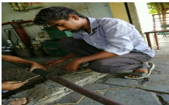
Fig. 4.2.3. Bolts are inserting into coinciding holes
