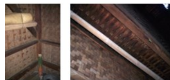
Fig. 10. Wall of Traditional House in Kampong Cikondang
