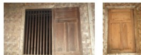
Fig. 11. Window of Traditional House in Kampong Cikondang
