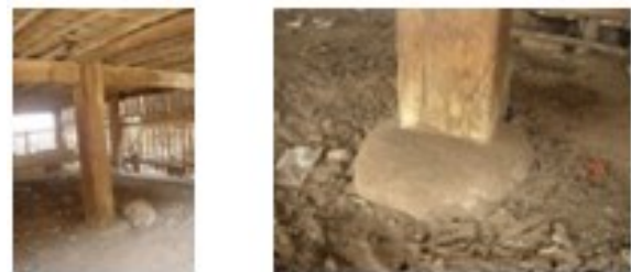
Fig. 4. Foundation of Traditional House in Kampong Panjalin
