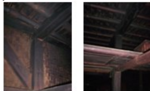
Fig. 9. Columns of Traditional House in Kampong Cikondang
