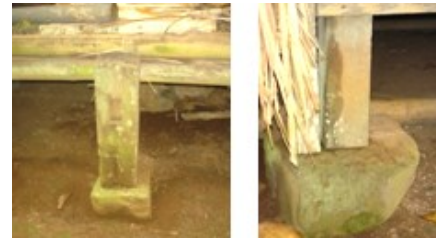
Fig. 8. Foundation of Traditional House in Kampong Cikondang
